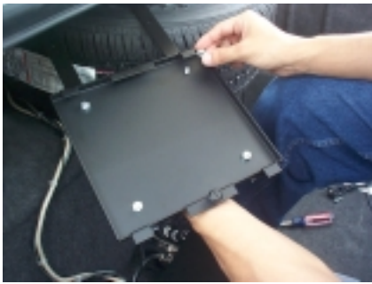
Assembly of the mounting brackets to the base plate of vault
