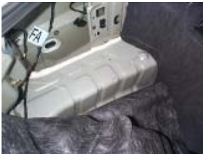
Partially remove carpet from work area.
